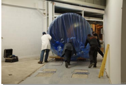
Figure 5: Installation of tube sections in the corridor.
